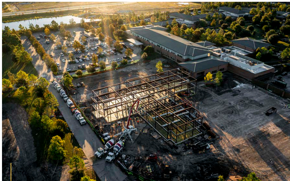
Construction of the Outpatient Services Center is underway and will be complete by July 2022. Menninger plans to establish The Center for Addiction Medicine and Recovery on the second floor.
